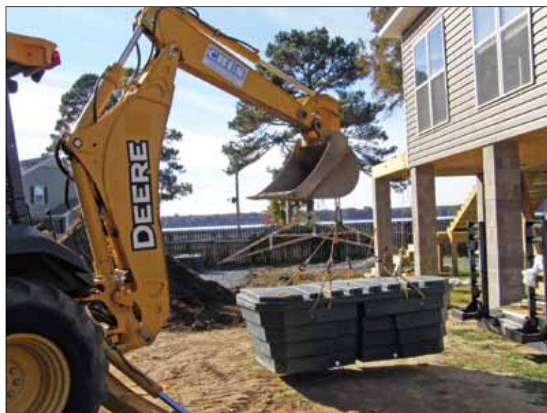
Brian Lucas of Lucas Soil Evaluation uses a John Deere backhoe to move a 150-gpd Puraflo peat biofilter. (Photos courtesy of Matt Vinson)
